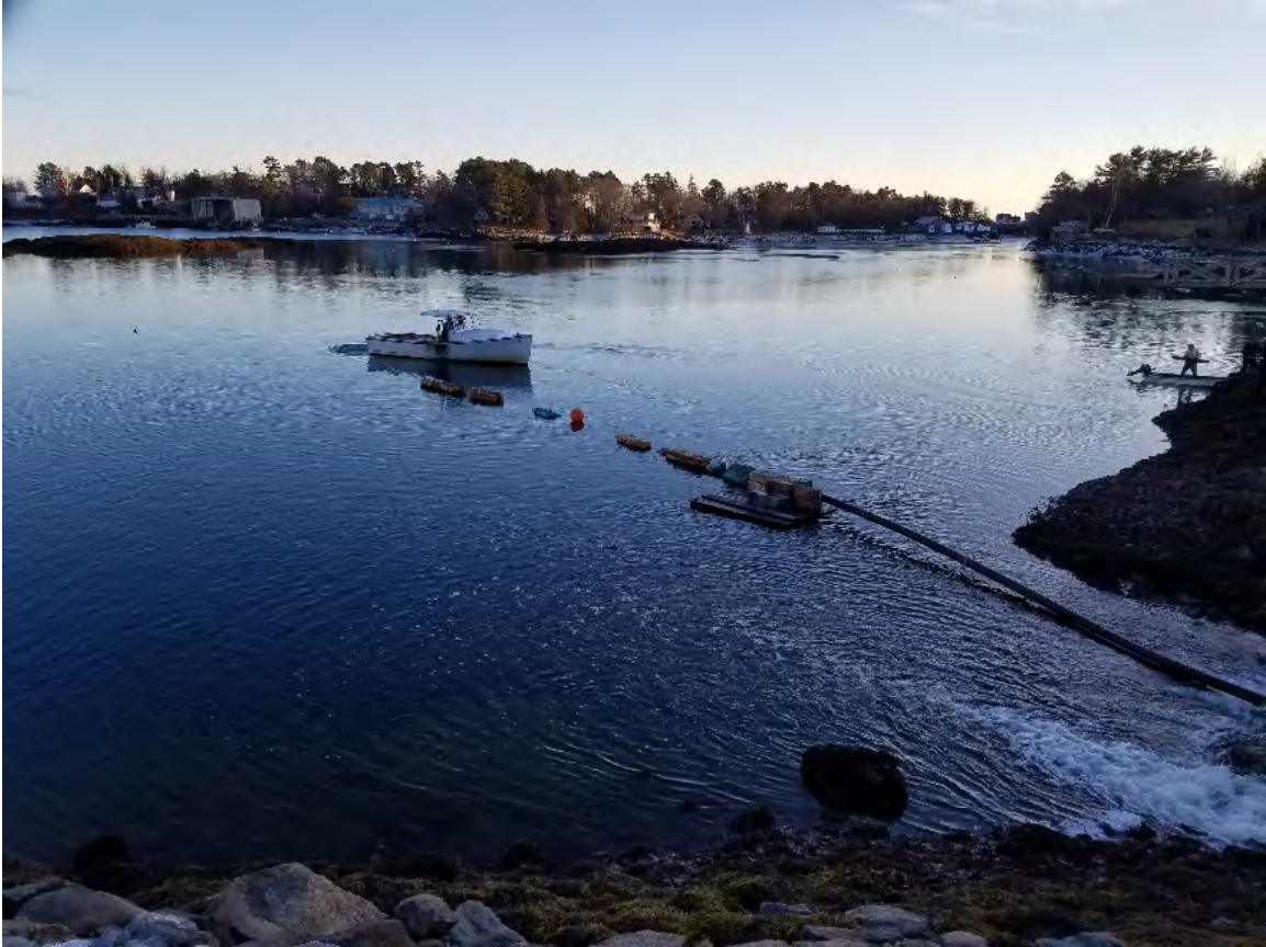
33: December 5 (end of the day): weights installed on half the length of the harbor-side siphon pipe
