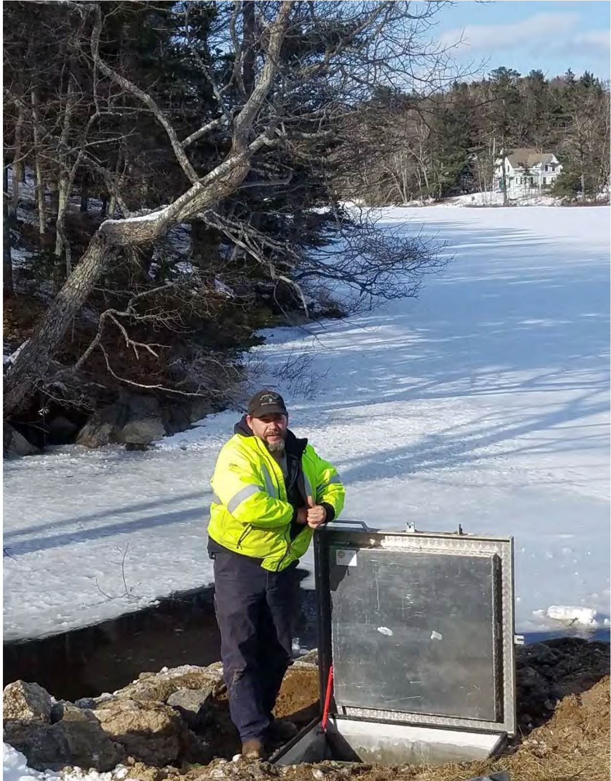
7: Dale Harmon, Operations Manager, Boothbay Region Water District, beside the manhole cylinder he and his crew assembled, after installation
