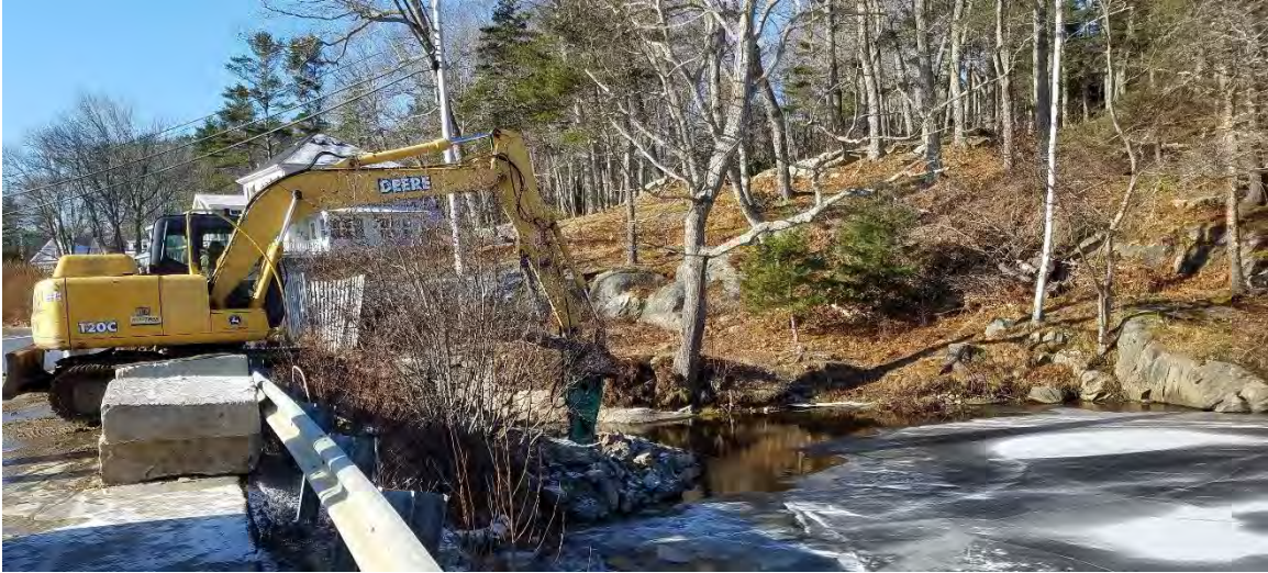
38: December 12: Hoe-ram removing ledge to gain the proper depth for the manhole cylinder
