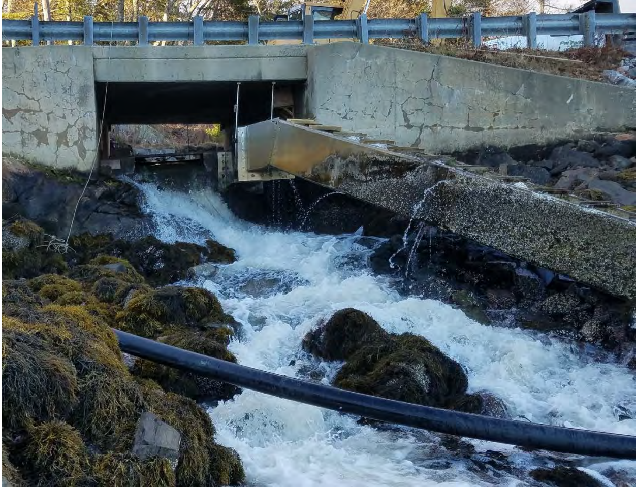
3: Box culvert and fishway as seen from harbor
