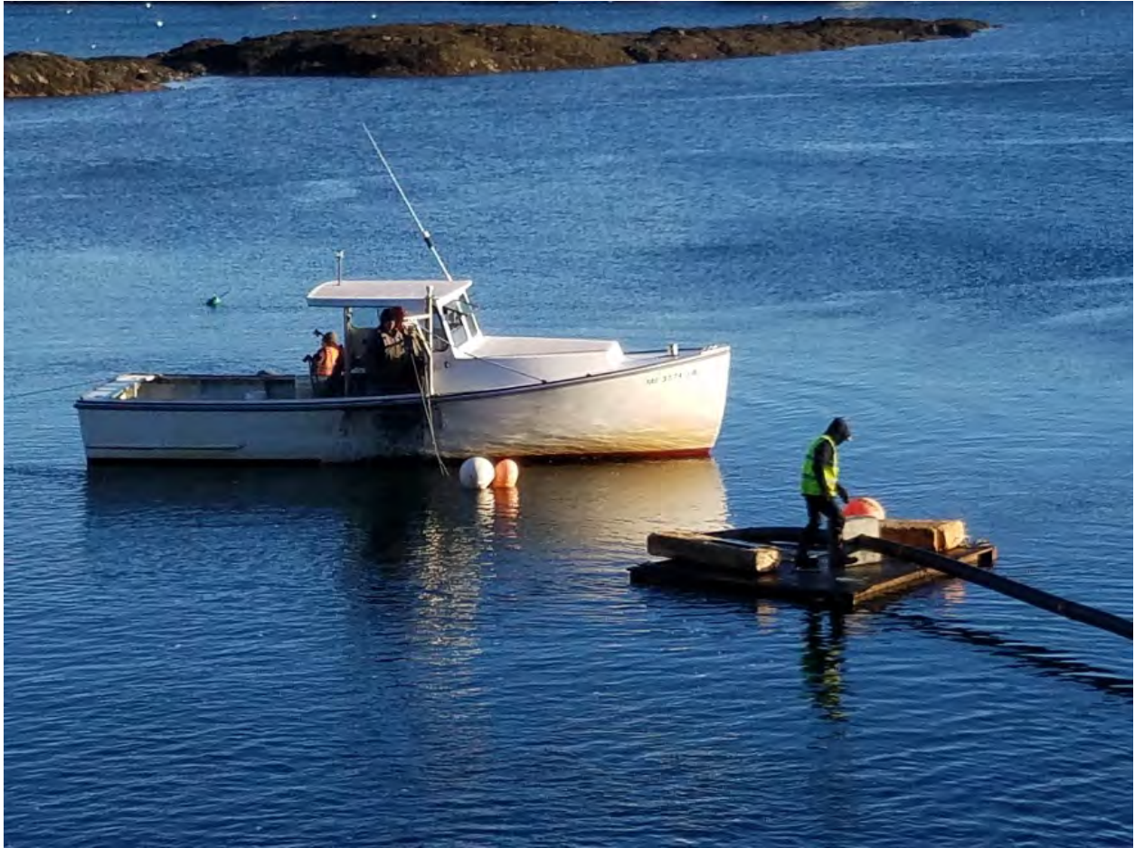
27: Kent in his lobster boat and Mike on work platform getting ready to place first weight on harbor-side siphon pipe
