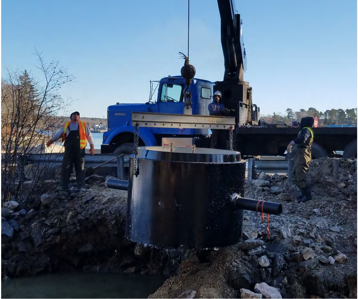
40: December 13: Crane lowering manhole cylinder into place
