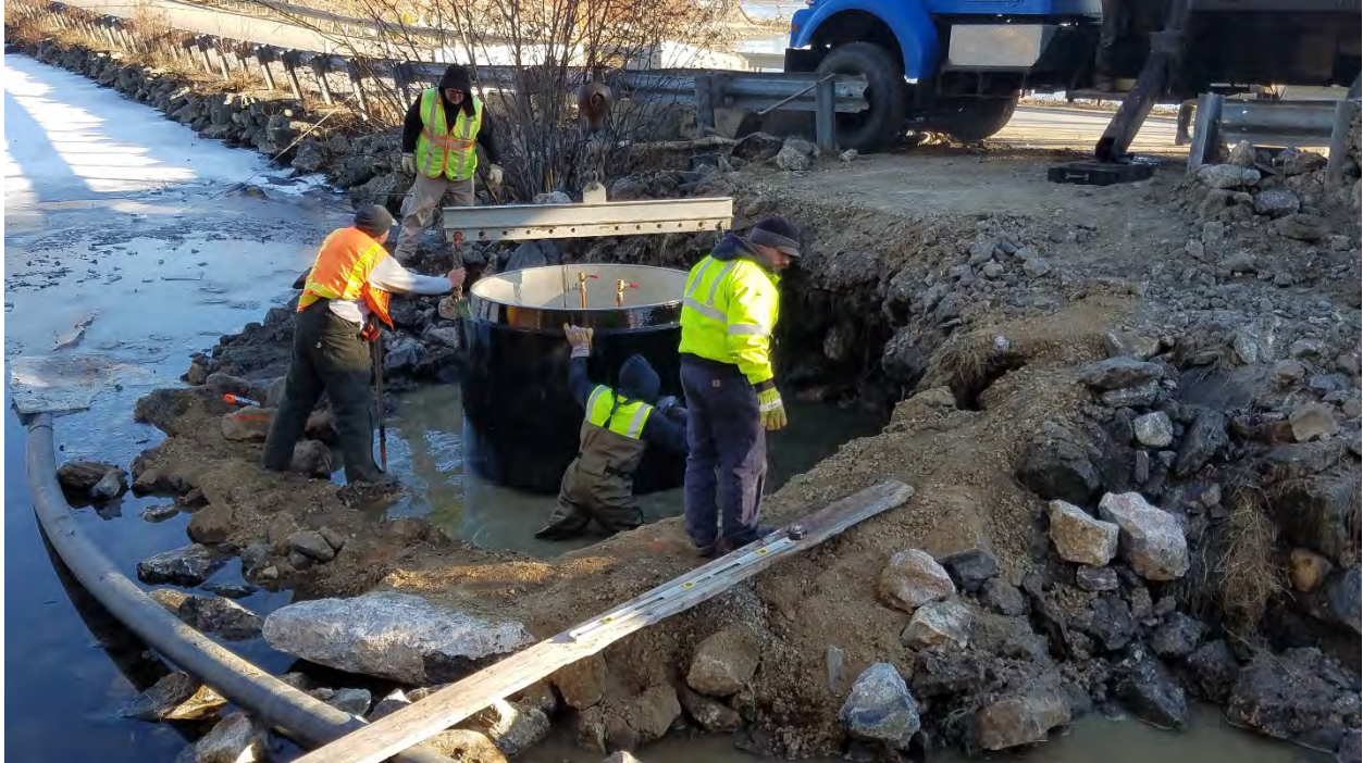
41: December 13: Manhole cylinder being lowered into place, Mike working hip-deep in frigid water
