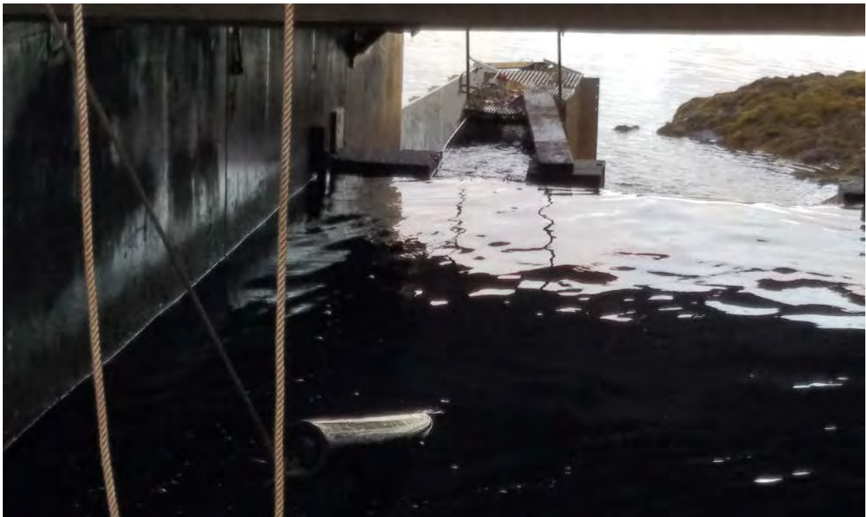
24: Siphon pipe emerging on pond side after being threaded through dam in box culvert
