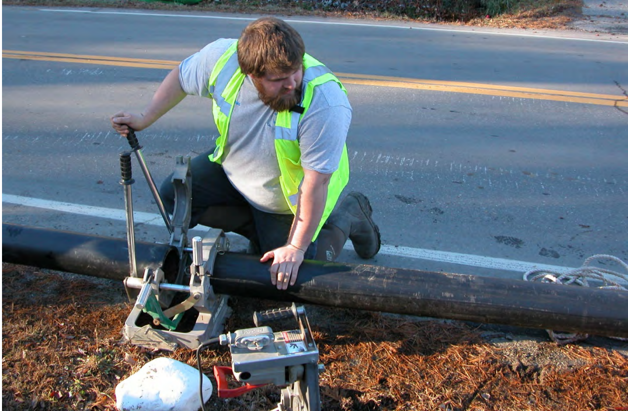
14: Shawn fusing two sections of pipe
