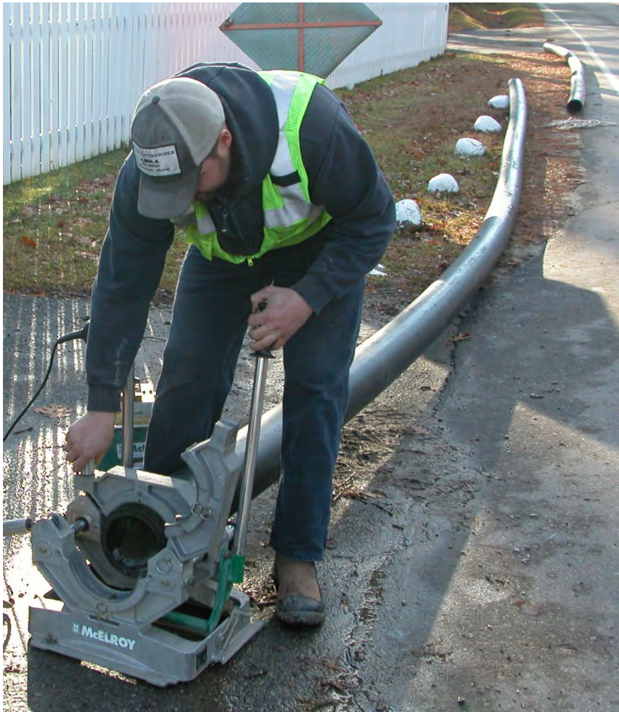
13: Taylor preparing the fusing apparatus
