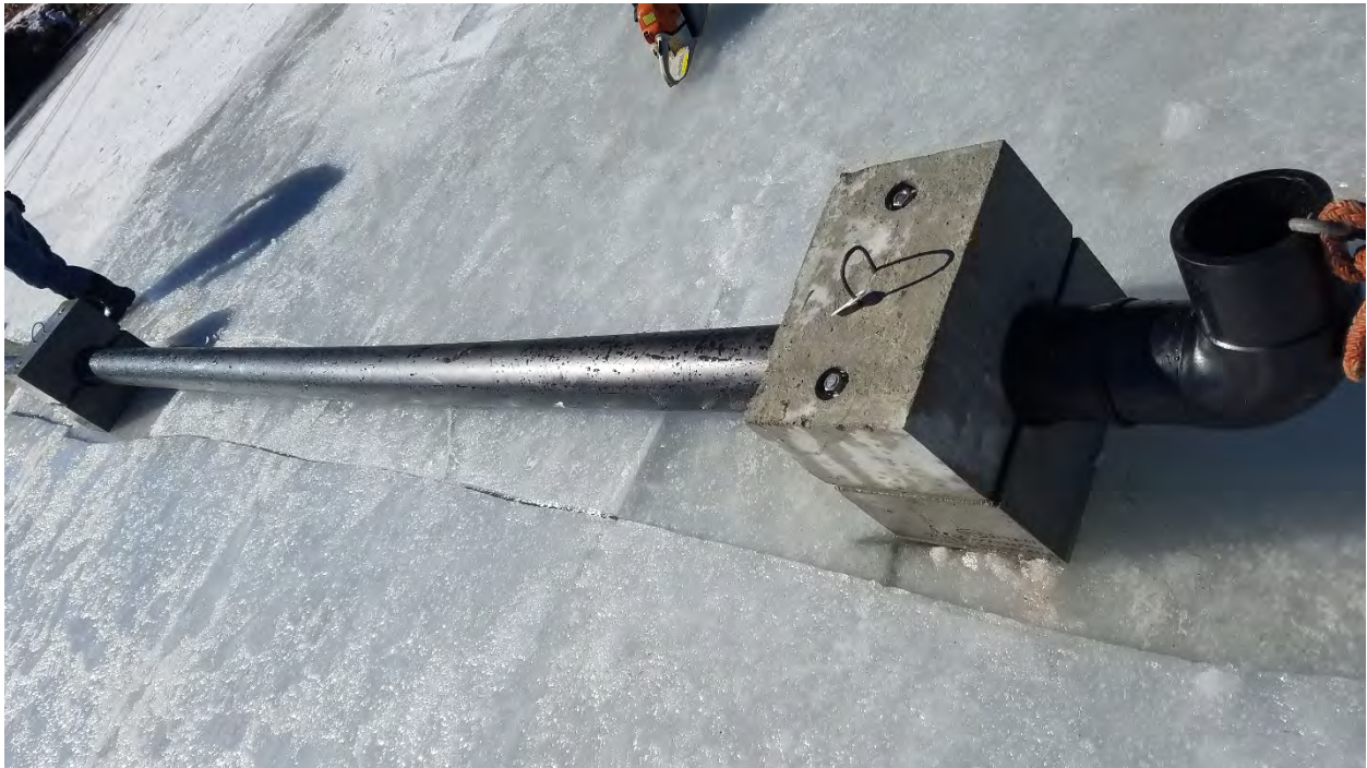
49: Even with the ice cut away beneath it, the siphon pipe was reluctant to take the plunge
