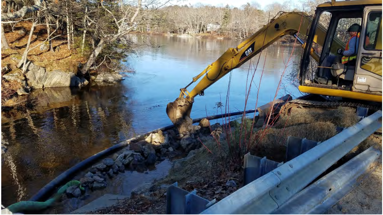
36: Preparing site for manhole cylinder
