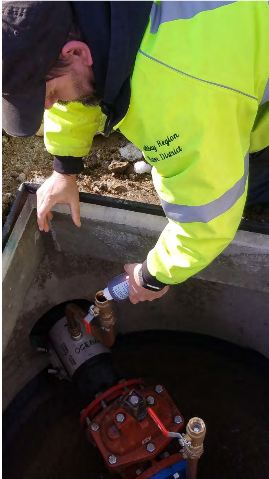
52: March 8: Dale Harmon placing tracing dye in the siphon
