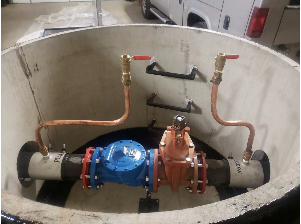
5: Controls for siphon, showing check valve (blue); large ball valve (orange) and two small ball valves
