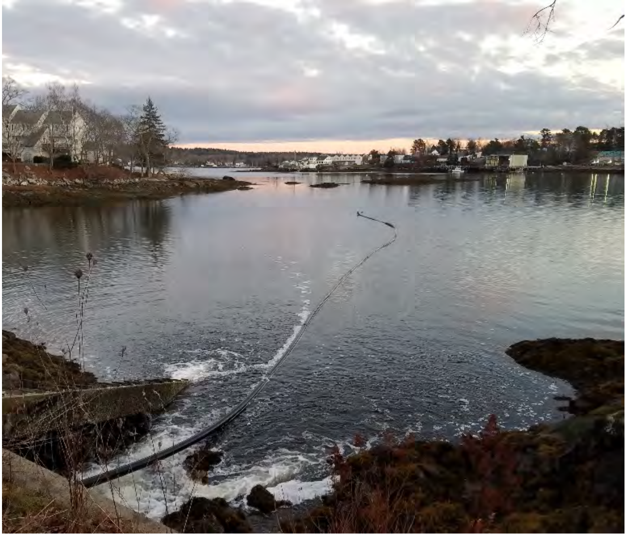
26: End of a long first day: the siphon pipe, filled with air, floating on surface of the harbor
