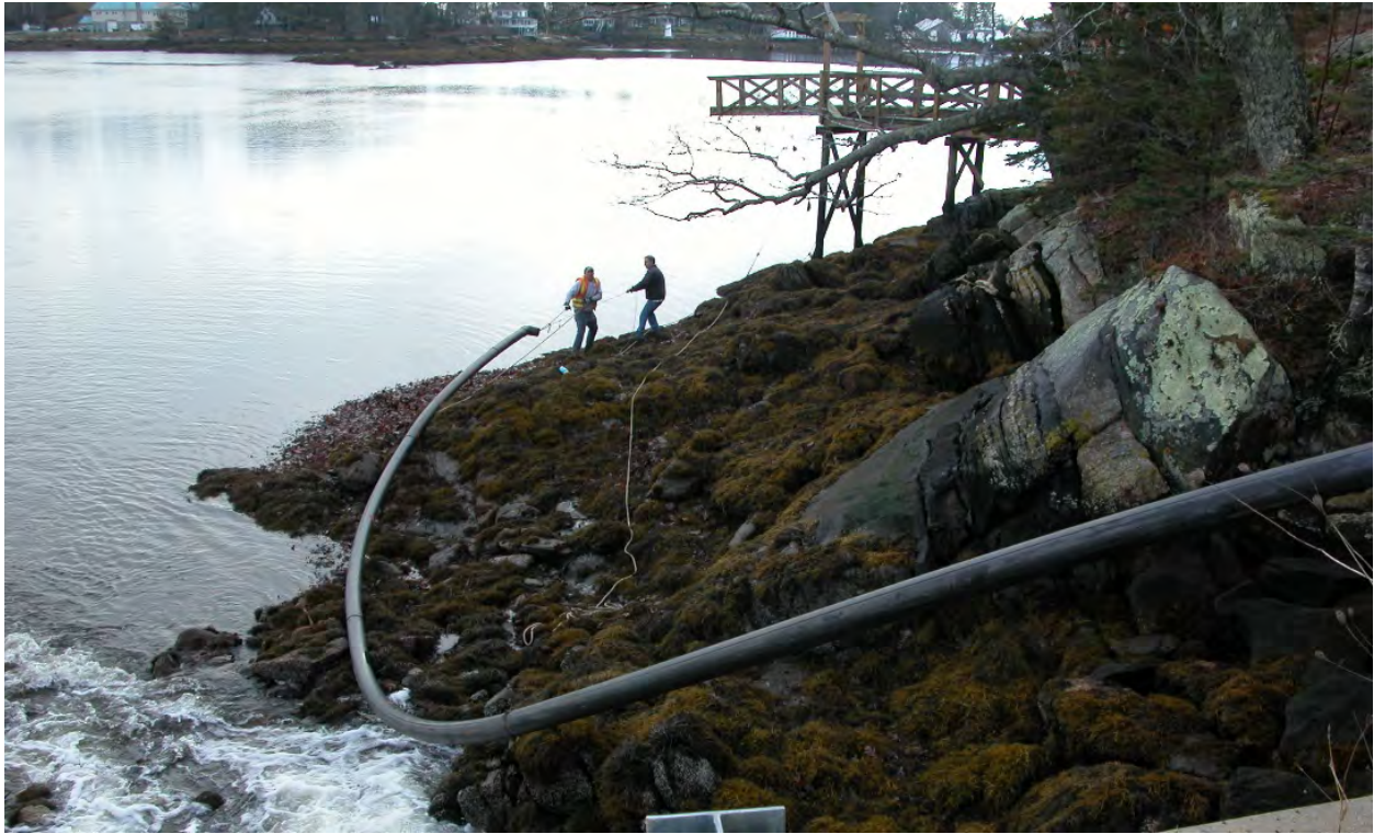
21: Kipp and Josh positioning the harbor-side siphon pipe for placement in the harbor
