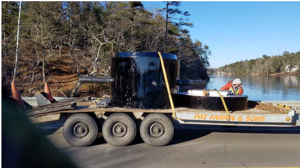
35: Manhole cylinder and top ready to be set in place
