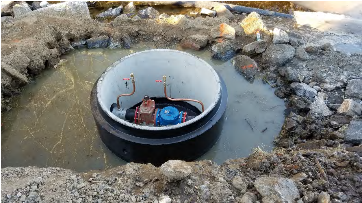
42: Manhole cylinder (without cover) in place
