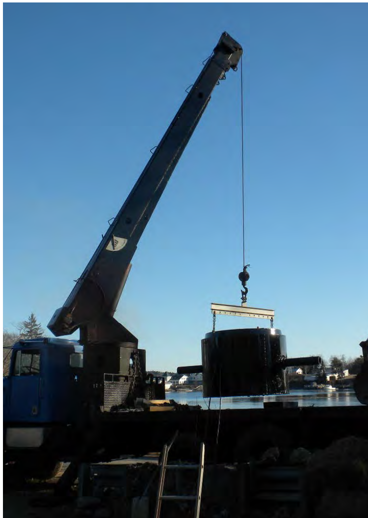
39: December 13: Crane lowering manhole cylinder into place
