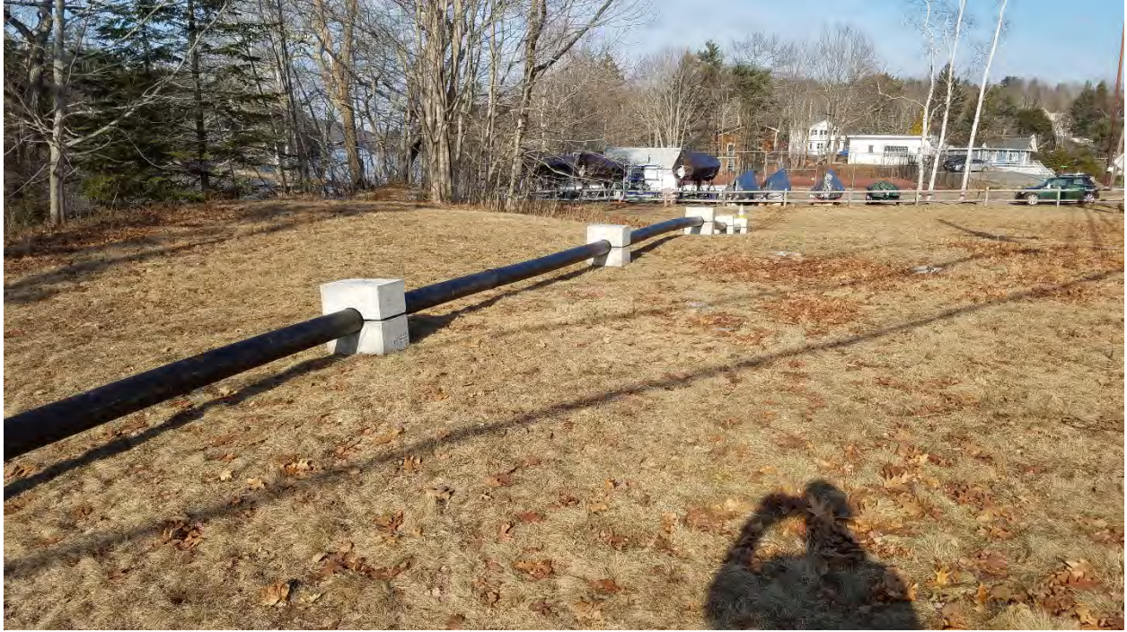
10: Pond-side siphon pipe with weights already attached
