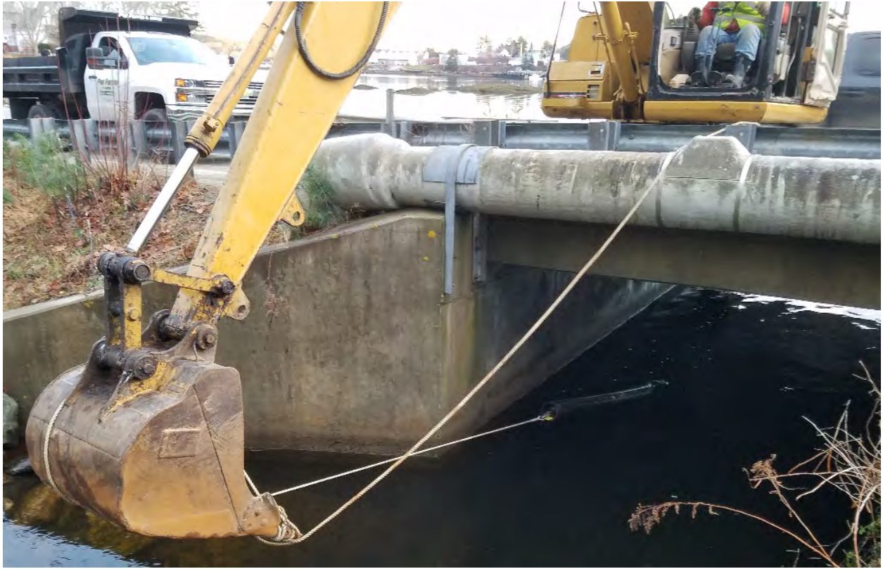
25: Siphon pipe being pulled through dam in box culvert
