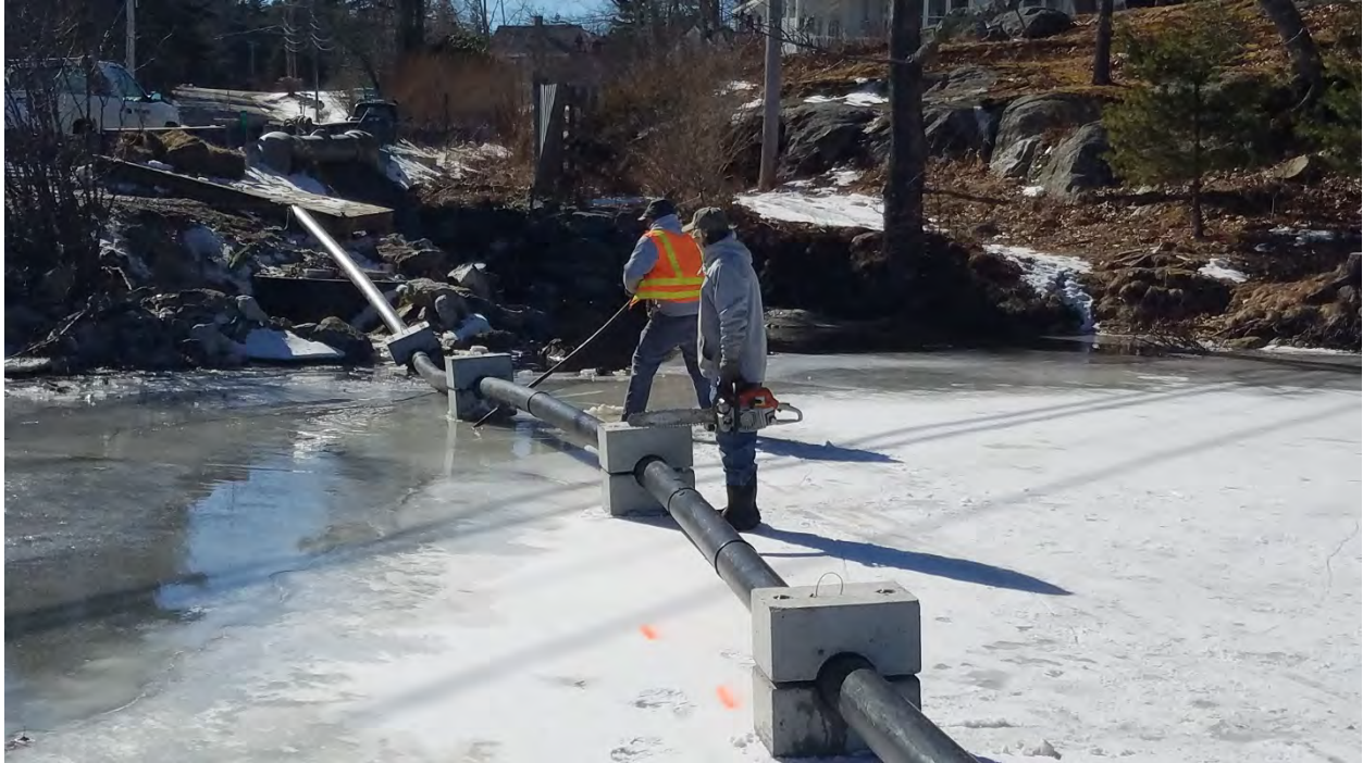
46: Kipp levering the pipe into the proper alignment
