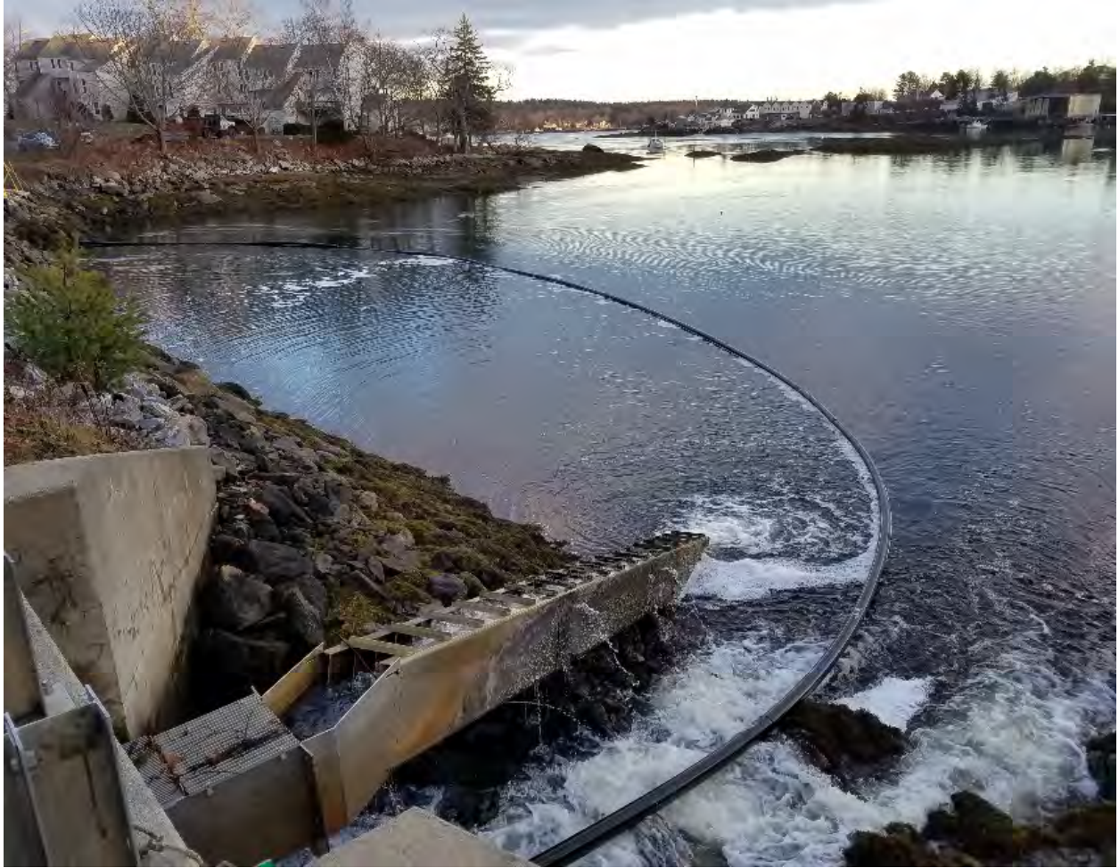
9: Harbor-side siphon pipe during installation (no weights attached yet)
