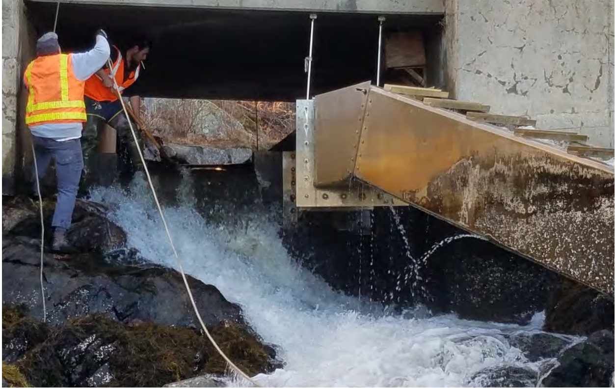
23: Kipp and Josh threading the siphon pipe through the dam in the box culvert
