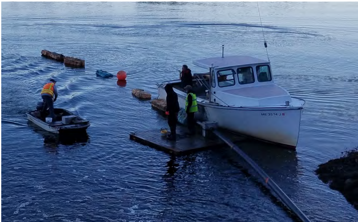
32: Installing weights on harbor-side siphon pipe continues
