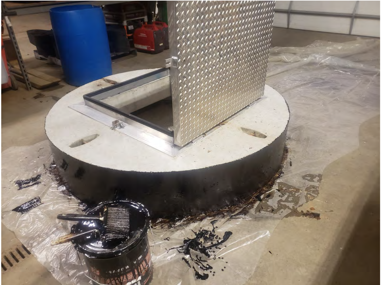
6: Manhole cylinder top (with hatch installed) being waterproofed at Water District workshop
