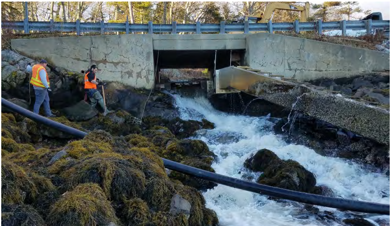
22: Kipp and Josh preparing to thread the siphon pipe through the dam in the box culvert
