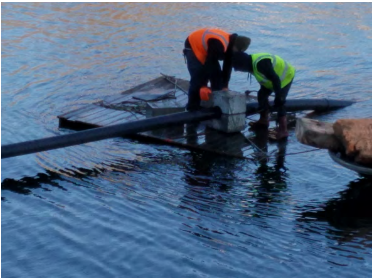
30: Mike and Josh wrestling the weighted siphon pipe off the work platform
