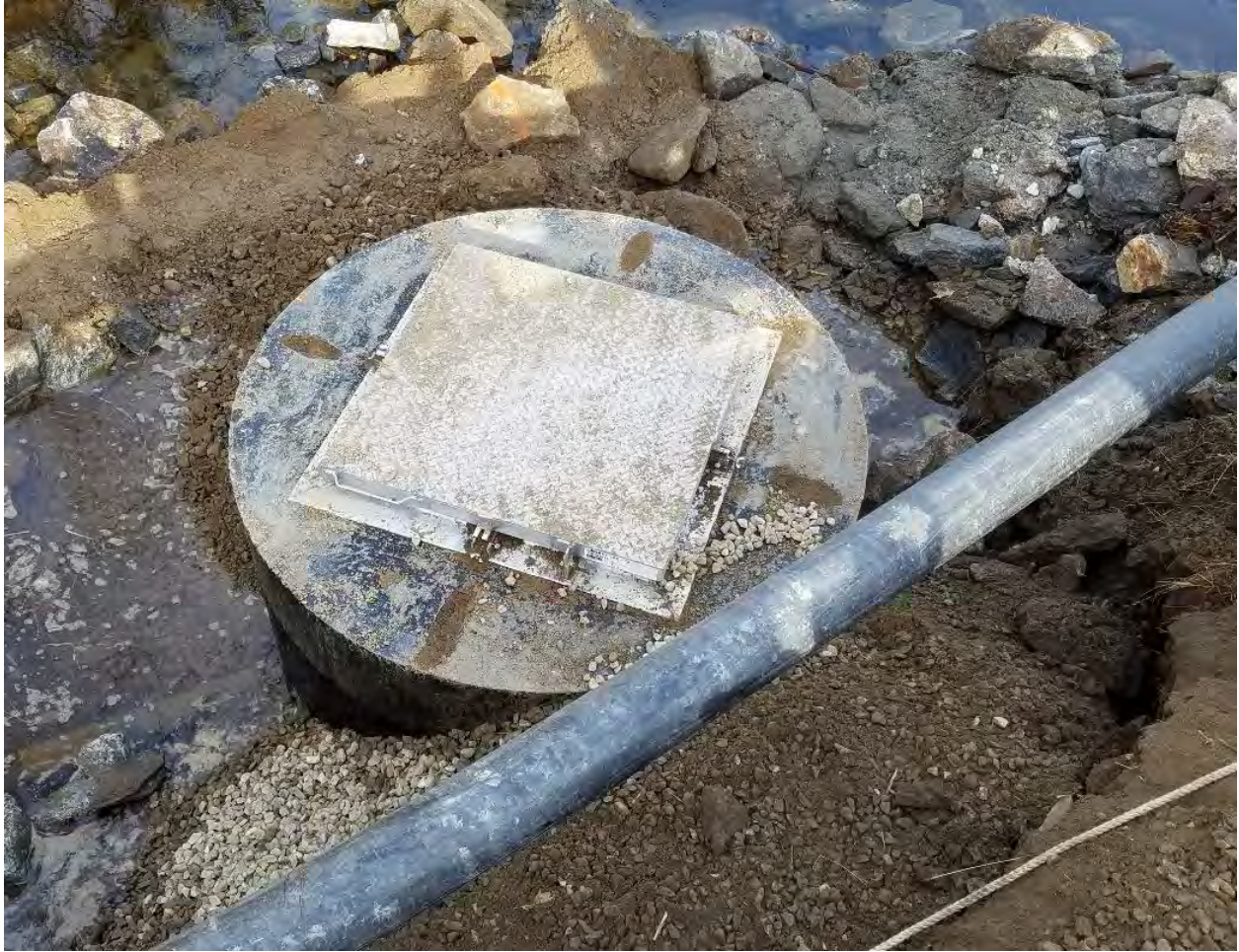
43: December 14: Manhole cylinder (with cover) in place; harbor-side siphon pipe awaiting attachment
