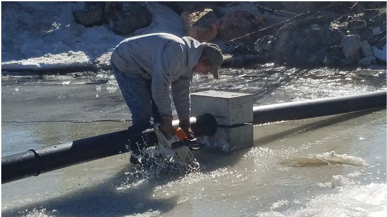
47: Mike cutting through the ice supporting the siphon pipe
