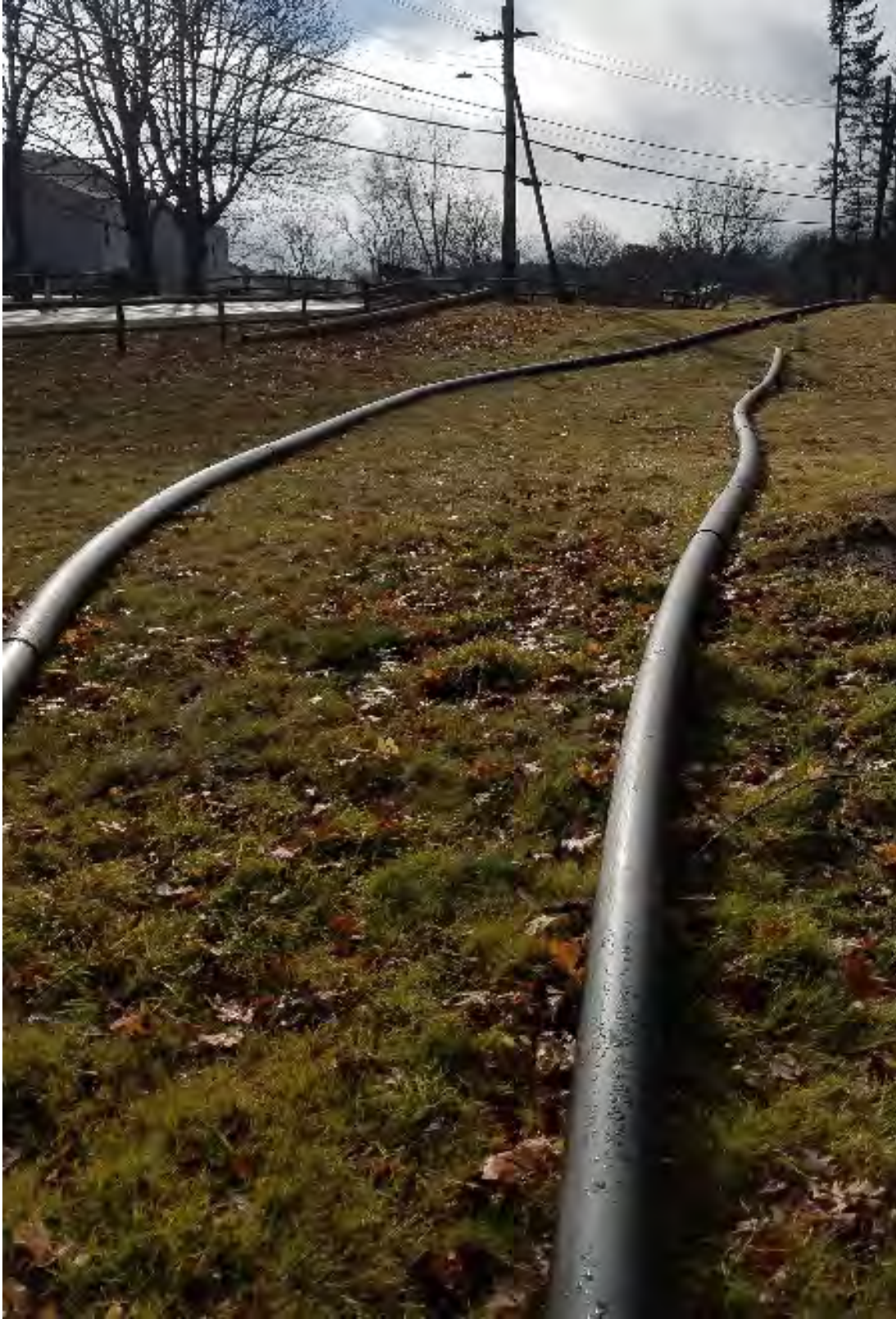
8: The two halves of the siphon pipe fused and ready for installation (150' and 100' respectively)
